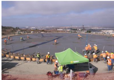
Construction of a new concrete reservoir (capacity of 3.4 million gallons) on Alta Rd.
